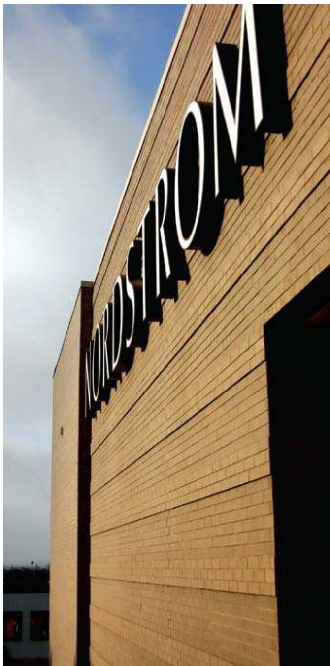
Fig. 6. With care and cooperation, consistent mortar color producing the appearance desired by the owner can be achieved.
