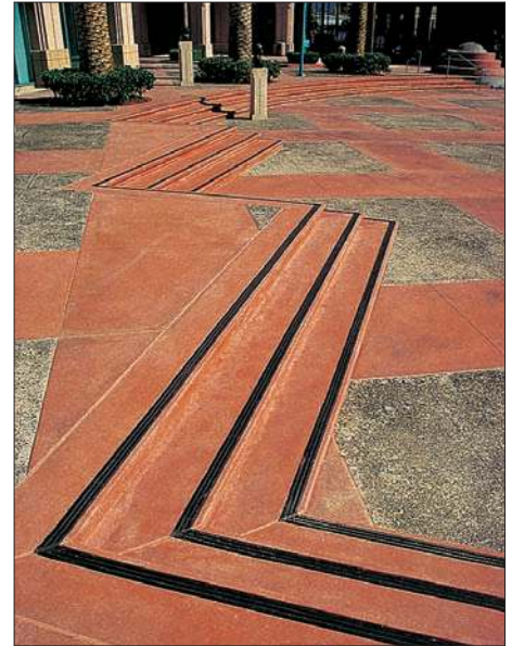
Integral color adds a design dimension to otherwise ordinary concrete.
