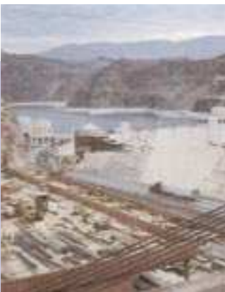
New visitor center rises from a V-cut in the canyon wall. Drum-shaped structure is clad with precast panels, some of which follow the profile of rocks and abut.
